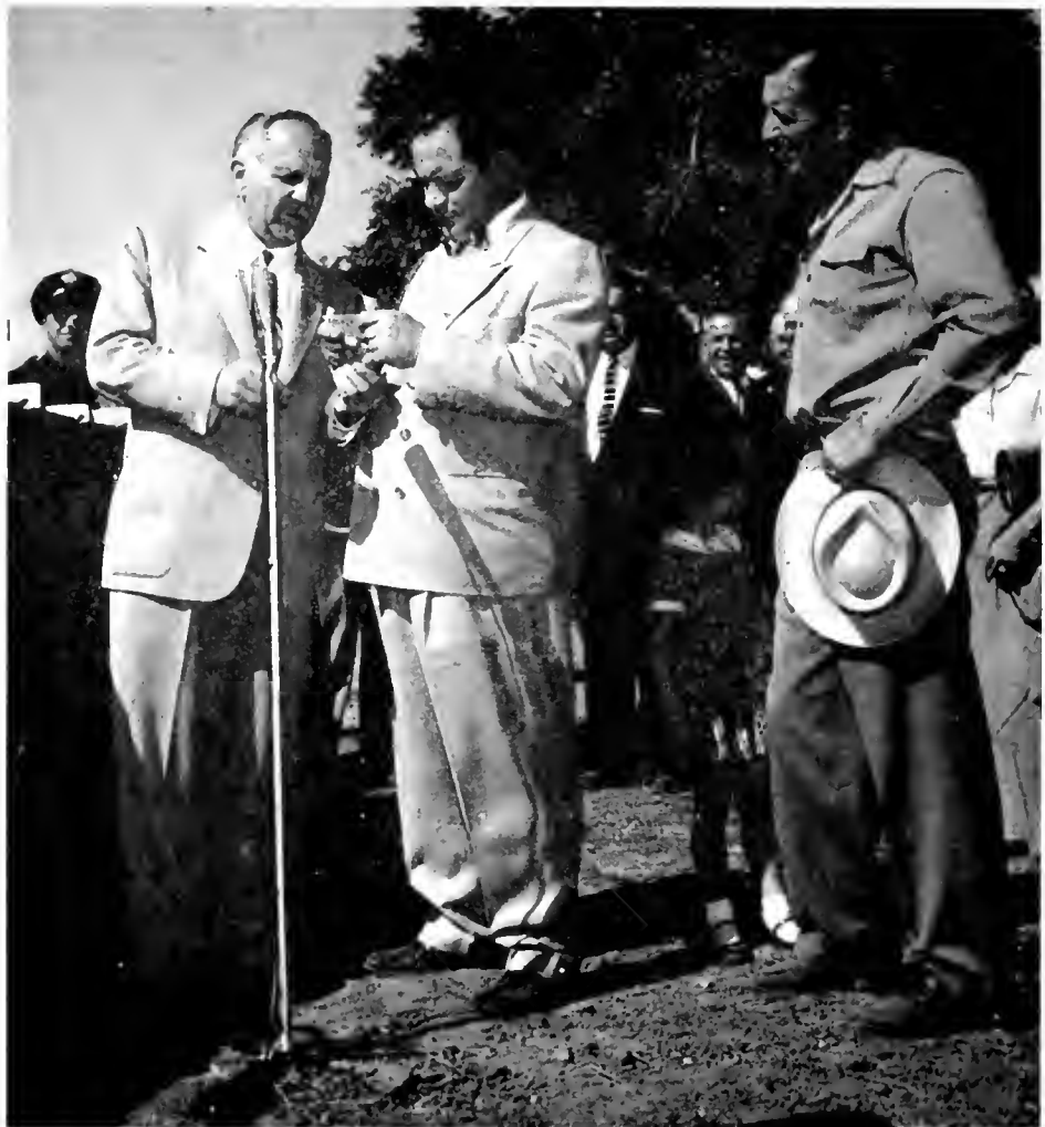
Rolph B. Bronson (center), business manager of the International Union of Operating Engineers, A.F.L., examines Governor Goodwin J. Knight's union membership card before the governor climbed aboard a bulldozer for groundbreaking ceremonies for an overhead crossing of Los Angeles' proposed Sepulveda Freeway. The card was in order. Looking on at right is Jock W. Baker, of Peterson and Baker, the contractors who will build the structure.
